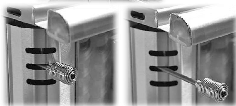
closed flue gas deflector (17)
